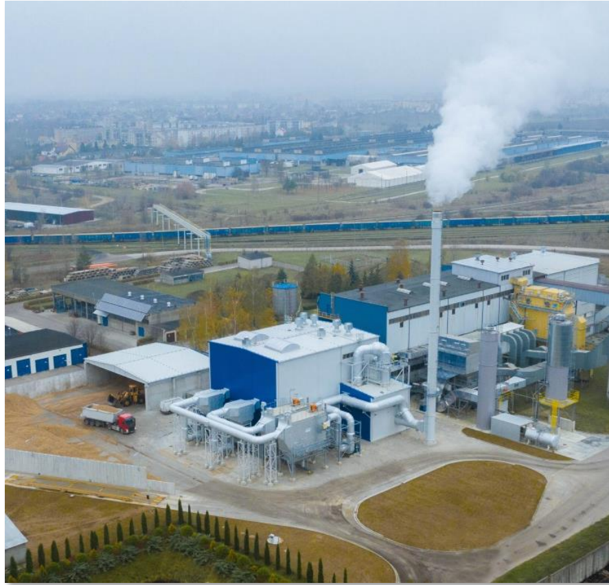
2x12 MW biomass boiler plant
