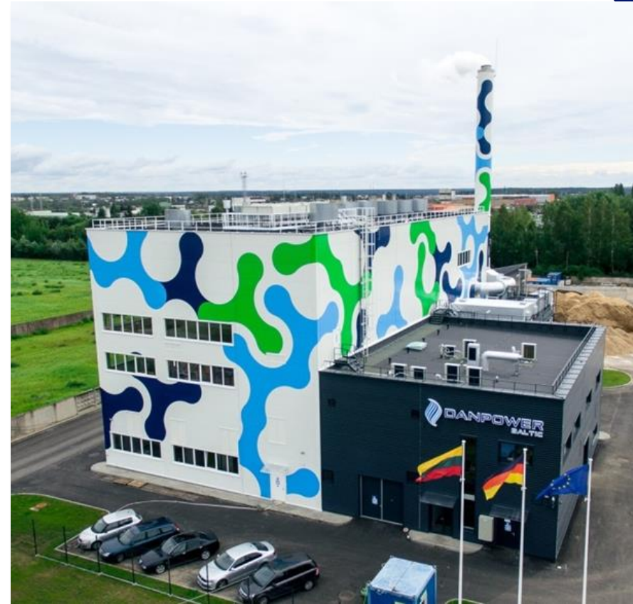
5 MWe biomass boiler plant Total capacity - 26,3 MW
