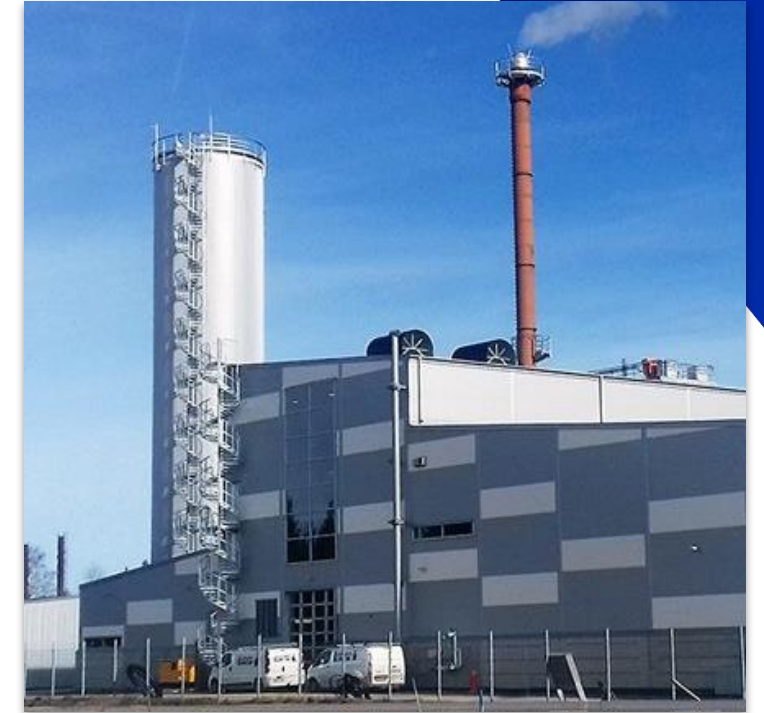
10,6 MW biomass boiler plant
