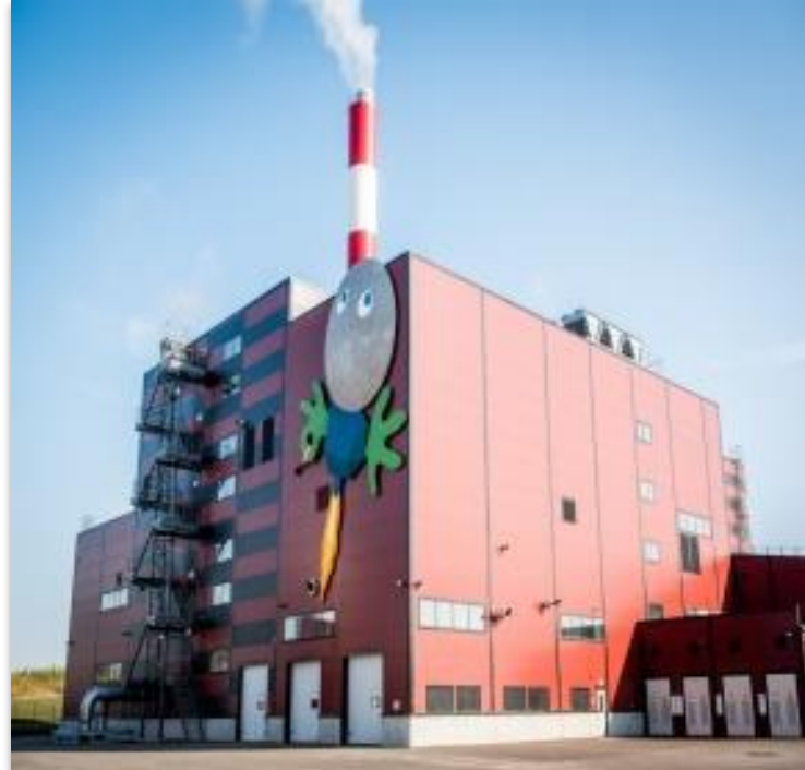
21 MWe biomass boiler plant Total capacity – 73,8 MW
